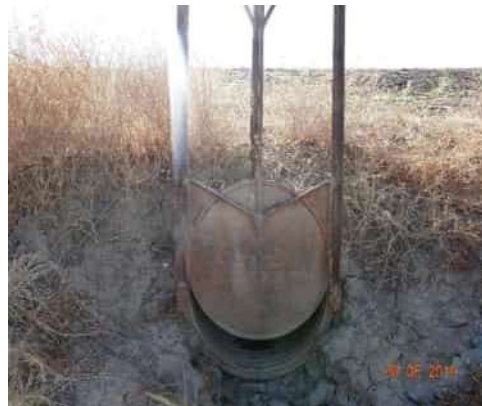
08/05/2019 (ST0003U01 LM:18.612) : WS view: close up of the slide gate.
