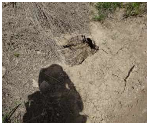
04/14/2016 (ST0003U01 LM:18.612) : WS slope: slight borrowing activity
