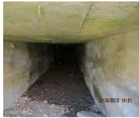
12/10/2012 (ST0003U01 LM:13.376) : LS view: inside concrete culvert
