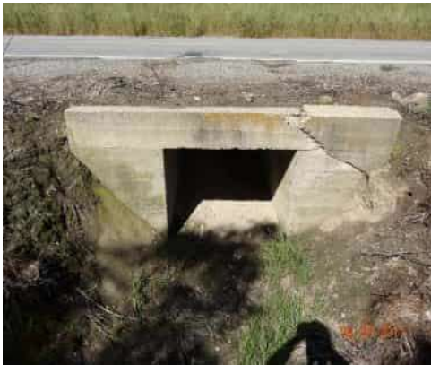
04/20/2017 (ST0003U01 LM:13.376) : LS headwall across River road.
