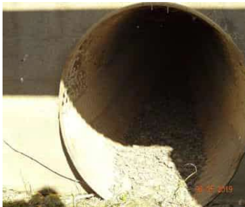
08/05/2019 (ST0003U01 LM:18.612) : LS view: pipe visible on LS.
