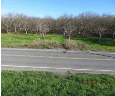
12/10/2012 (ST0003U01 LM:13.376) : LS view: overview of county road
