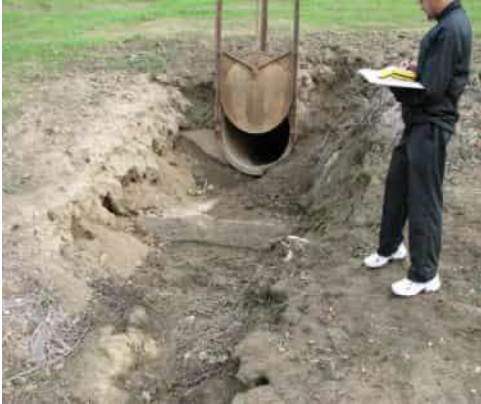
11/27/2012 (ST0003U01 LM:18.612) : WS view: outlet pipe with concrete headwall and floor apron.
