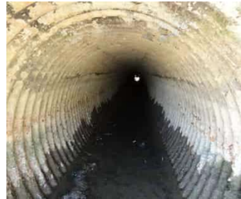
04/14/2016 (ST0003U01 LM:12.963) : LS view: inside CMP outlet with some water in it.
