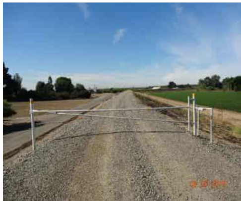
08/05/2019 (ST0003U01 LM:18.612) : Overview of levee crown looking d/s towards pipe crossing.
