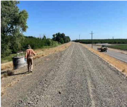
06/13/2024 (ST0003U01 LM:13.376) : View of levee crown
