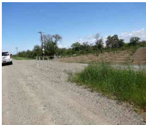
04/14/2016 (ST0003U01 LM:13.376) : Looking upstream from crown and facing LS.
