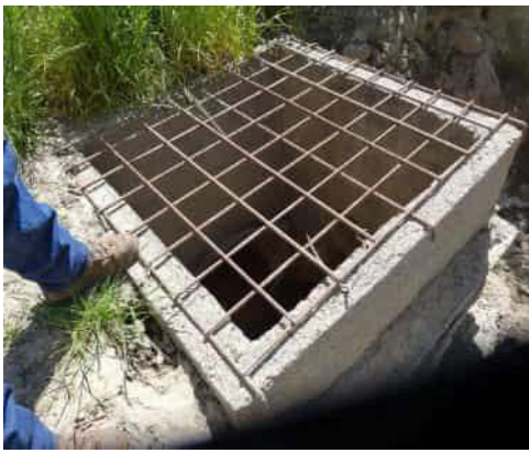
04/14/2016 (ST0003U01 LM:12.963) : WS slope: pipe visible inside concrete surge box (photo taken facing WS slope)
