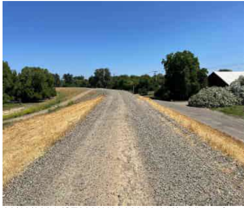
06/13/2024 (ST0003U01 LM:18.612) : View of crown
