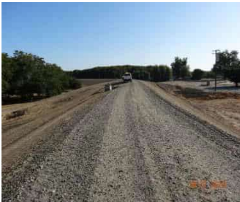
11/12/2019 (ST0003U01 LM:12.963) : Overview of levee crown looking u/s towards pipe crossing.
