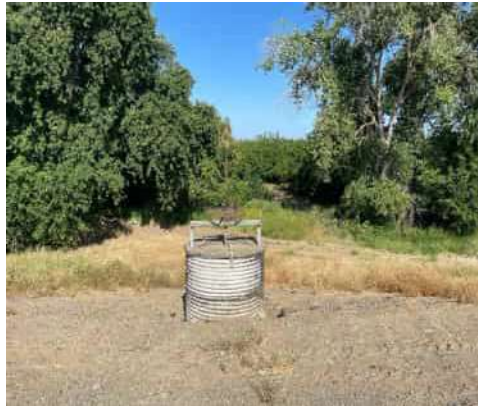
06/13/2024 (ST0003U01 LM:13.376) : View of waterside with CMP riser
