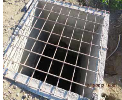
12/10/2012 (ST0003U01 LM:12.963) : WS view: concrete surge box
