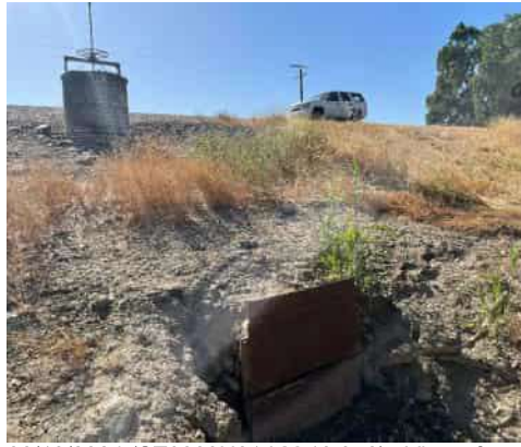
06/13/2024 (ST0003U01 LM:13.376) : View of capped pipe on WS
