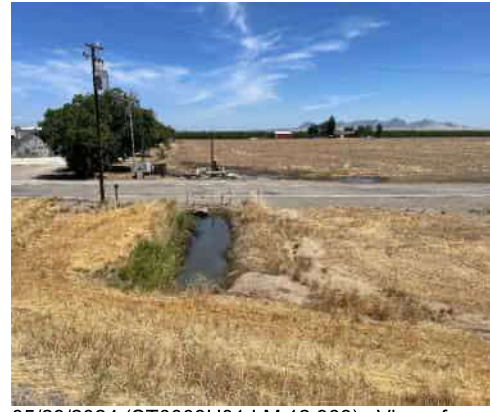
05/29/2024 (ST0003U01 LM:12.963) : View of landside
