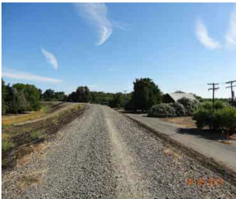
08/05/2019 (ST0003U01 LM:18.612) : Overview of levee crown looking u/s towards pipe crossing.
