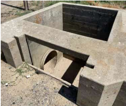
06/13/2024 (ST0003U01 LM:18.612) : View of pipe in distribution box on landside
