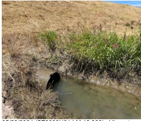
05/29/2024 (ST0003U01 LM:12.963) : View at landside pipe opening
