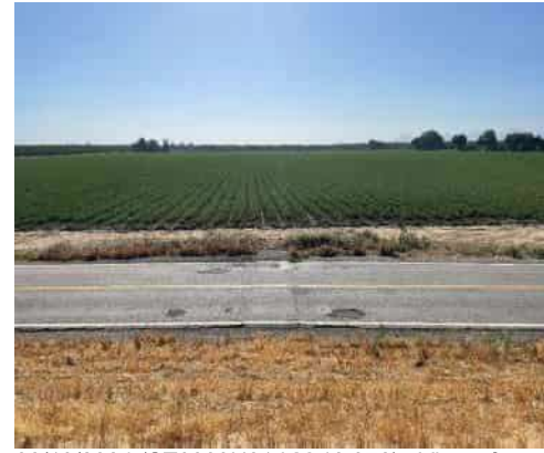
06/13/2024 (ST0003U01 LM:13.376) : View of landside
