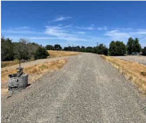
05/29/2024 (ST0003U01 LM:12.963) : View of levee crown
