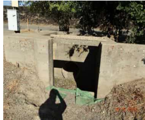
08/05/2019 (ST0003U01 LM:18.612) : LS view: concrete structure located on LS.
