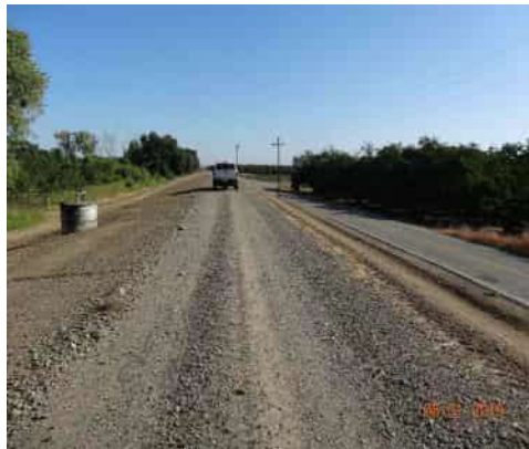
08/01/2019 (ST0003U01 LM:13.376) : Overview of levee crown looking u/s towards pipe crossing.
