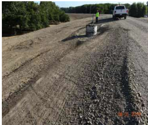
11/12/2019 (ST0003U01 LM:12.963) : WS view: CMP riser located on WS slope.
