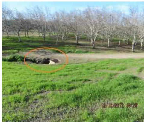
12/10/2012 (ST0003U01 LM:12.963) : WS view: overview of concrete surge box
