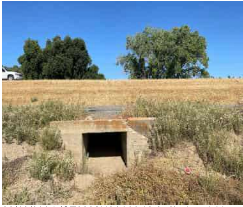
06/13/2024 (ST0003U01 LM:13.376) : Landside pipe end
