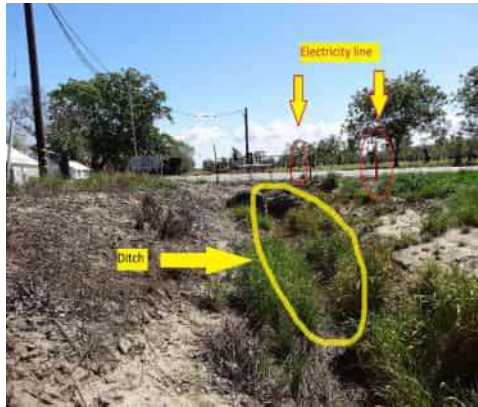
04/14/2016 (ST0003U01 LM:12.963) : LS view of unlined ditch with water in it. (Electricity line runs parallel to levee toward solar panels)
