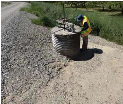
04/14/2016 (ST0003U01 LM:12.963) : WS slope: riser with slide gate. Erosion around riser cited during previous visit appears to be fixed.
