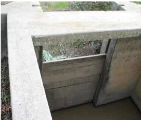
11/27/2012 (ST0003U01 LM:18.612) : LS view: wooden gate at inlet box.
