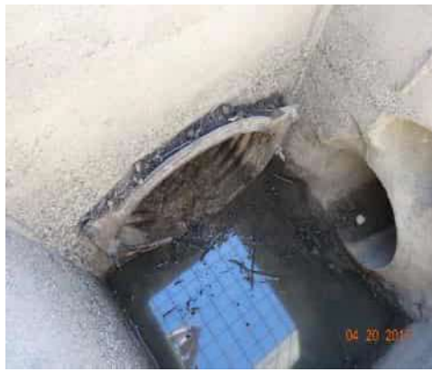
04/20/2017 (ST0003U01 LM:12.963) : View inside of WS surge box 4/20/2017
