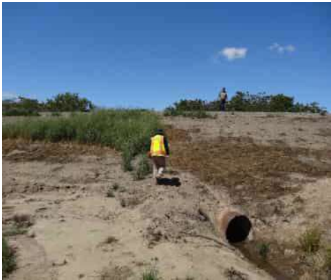
04/14/2016 (ST0003U01 LM:12.963) : View of LS slope above ditch.
