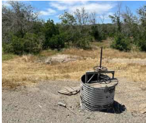
05/29/2024 (ST0003U01 LM:12.963) : View of waterside and CMP riser
