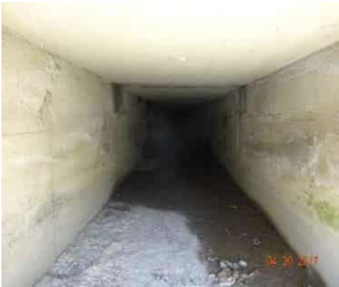
04/20/2017 (ST0003U01 LM:13.376) : View inside LS pipe end
