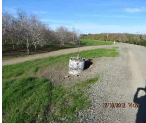
12/10/2012 (ST0003U01 LM:12.963) : WS view: CMP riser on levee slope.
