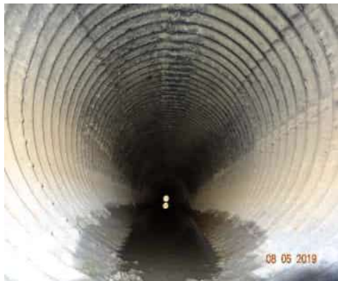
08/05/2019 (ST0003U01 LM:18.612) : WS view: inside view of pipe from WS.
