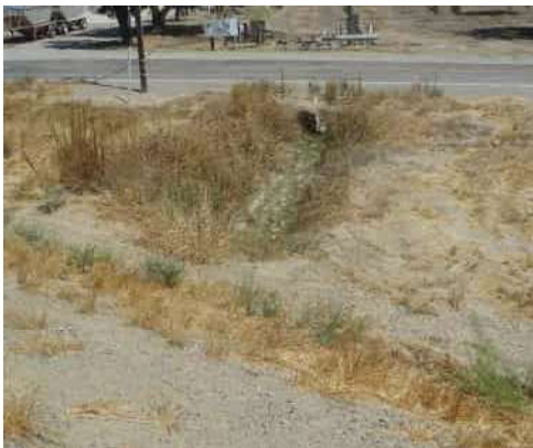
08/30/2018 (ST0003U01 LM:12.963) : LS view: ditch looks same as last inspection.
