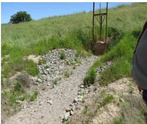
04/14/2016 (ST0003U01 LM:18.612) : WS slope: rock revetment placed along slide gate to repair sloughing.
