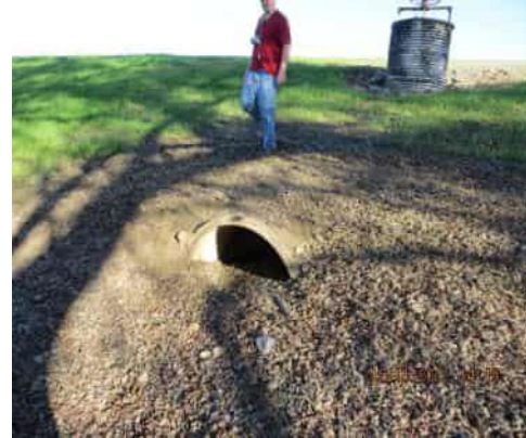
12/10/2012 (ST0003U01 LM:13.376) : WS view: overview of CMP riser and outlet pipe
