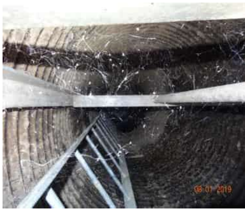
11/12/2019 (ST0003U01 LM:12.963) : WS view: inside view of CMP riser.
