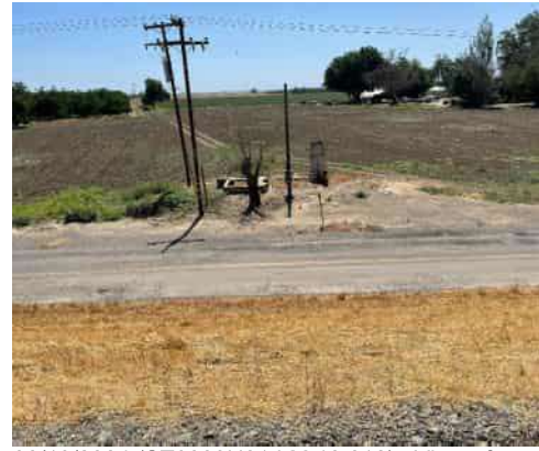
06/13/2024 (ST0003U01 LM:18.612) : View of landside and distribution box
