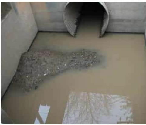
11/27/2012 (ST0003U01 LM:18.612) : LS view: soil deposite in inlet box
