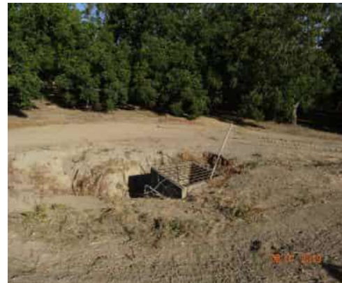
11/12/2019 (ST0003U01 LM:12.963) : WS view: concrete vault with screen located on the WS toe.
