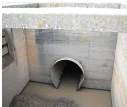
11/27/2012 (ST0003U01 LM:18.612) : LS view: inlet structure
