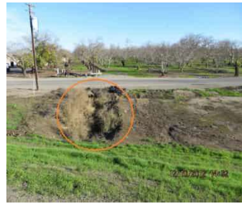
12/10/2012 (ST0003U01 LM:12.963) : LS view: overview of ditch
