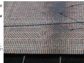
12 A119 OPEN MORTAR JOINTS SCALE: NOT TO SCALE REF: A110
