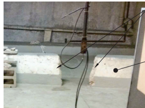
1 A118 DAMAGED CONCRETE
