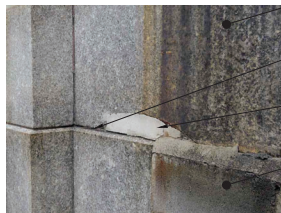
14 A118 DAMAGED GRANITE
