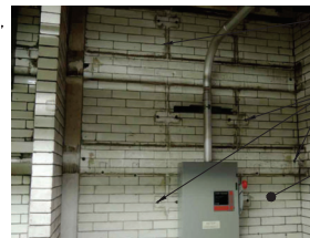
7 A118 DAMAGED BRICK
