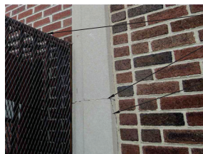
1 A119 CRACKED SURROUND SCALE: NOT TO SCALE REF: A110
