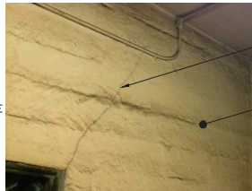
2 A118 CRACKED CONCRETE
