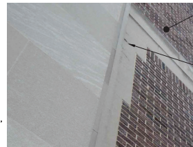
11 A118 CRACKED LIMESTONE
