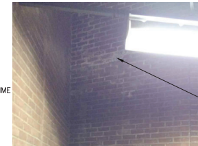
4 A118 EFFLORESCENCE
