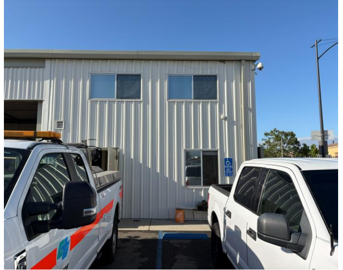
Electrical Office_1 (three windows & screen)
