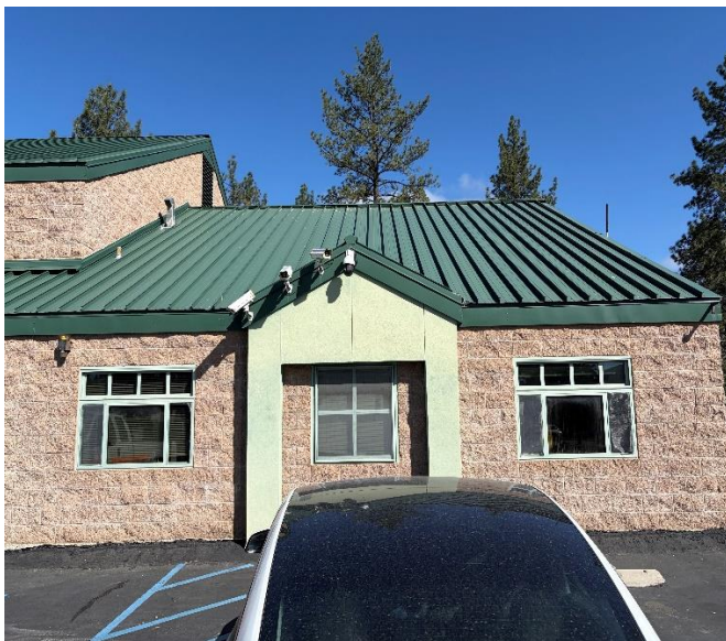
Office_1 (three windows & Screen)
