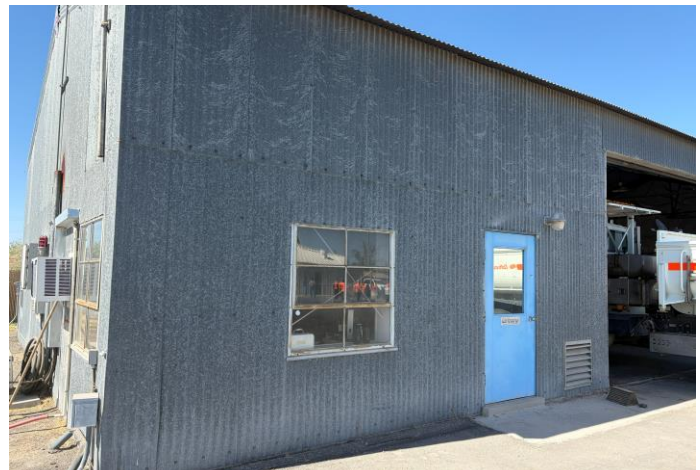
Equipment shop_1 ( one window & Screen)
