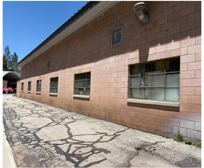
Equipment shop_1 (six windows: no sliding)
