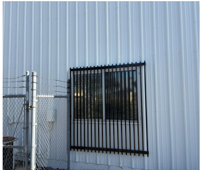
Electrical Office_3 (one window & screen)
