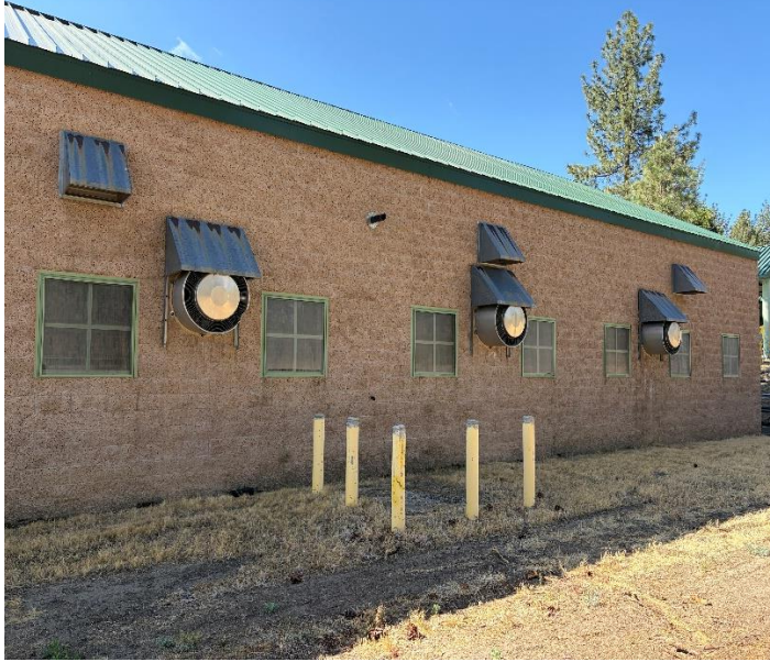
Equipment shop_1 (seven windows & sliding)
