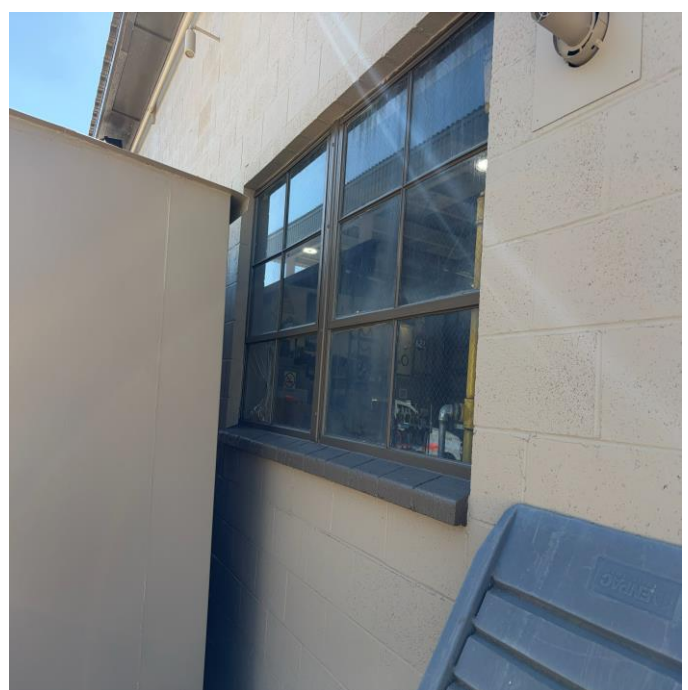
Equipment shop_1 (one window for repair)
