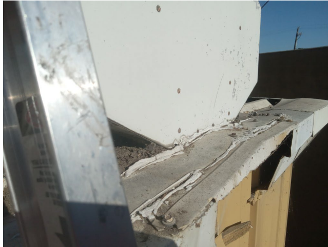
Photo 10 – 1334 West Fremont Street building roof penetration mastic.
