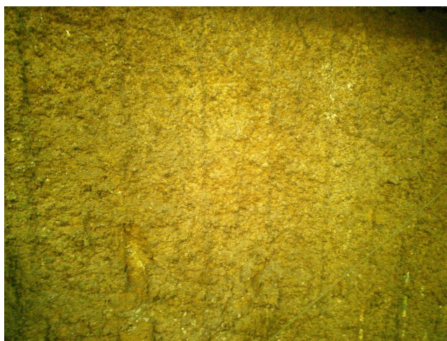
Photo 14 – 1326 West Fremont Street building spray insulation.
