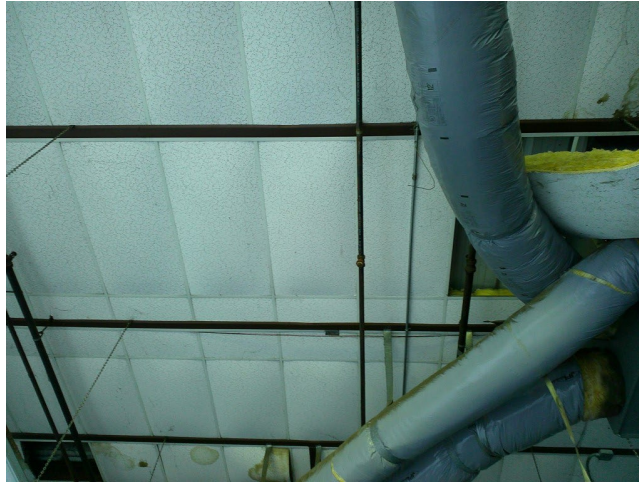
Photo 4 – 1414 West Fremont Street building fiberglass insulation and ducting.
