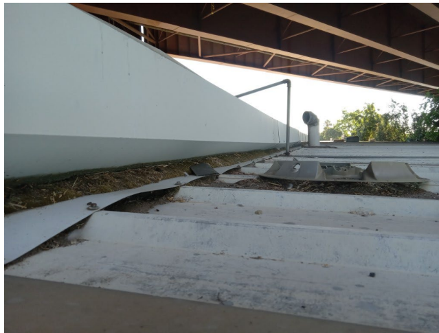
Photo 17 – 1326 West Fremont Street building roof penetration mastic.
