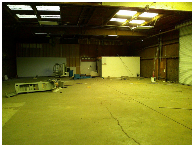
Photo 13 – 1326 West Fremont Street building in Stockton, San Joaquin County, California. Drywall/joint compound, wall texture, concrete slab, spray insulation and fiberglass insulation.
