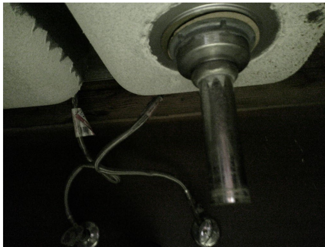
Photo 11 – 1334 West Fremont Street building sink undercoat.
