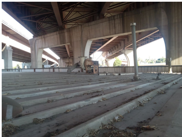
Photo 6 – 1414 West Fremont Street building roof penetration mastic.
