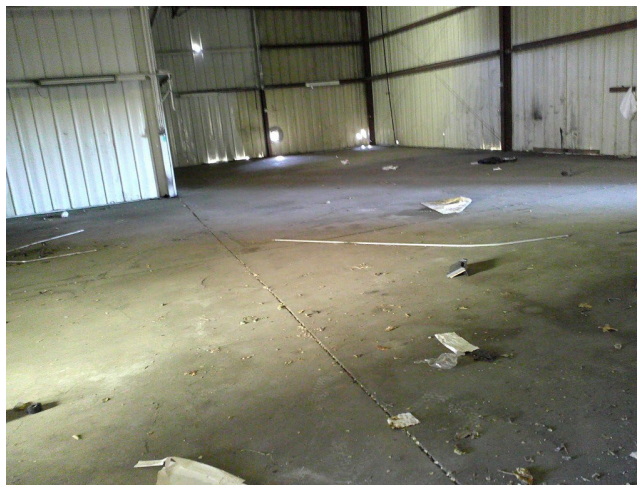
Photo 9 – 1334 West Fremont Street building concrete slab.
