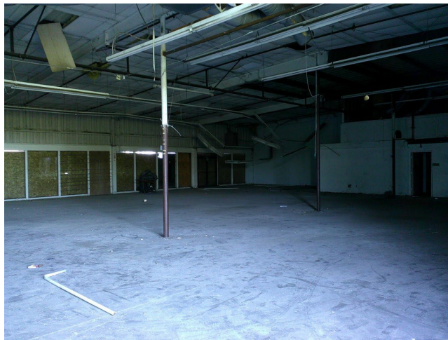
Photo 2 – 1414 West Fremont Street building drywall/joint compound, wall texture, acoustic ceiling panels, concrete slab and fiberglass insulation.
