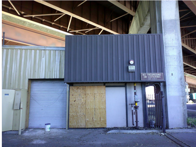
Photo 1 – 1414 West Fremont Street building in Stockton, San Joaquin County, California.
