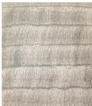
Proper Coverage on Insulation
