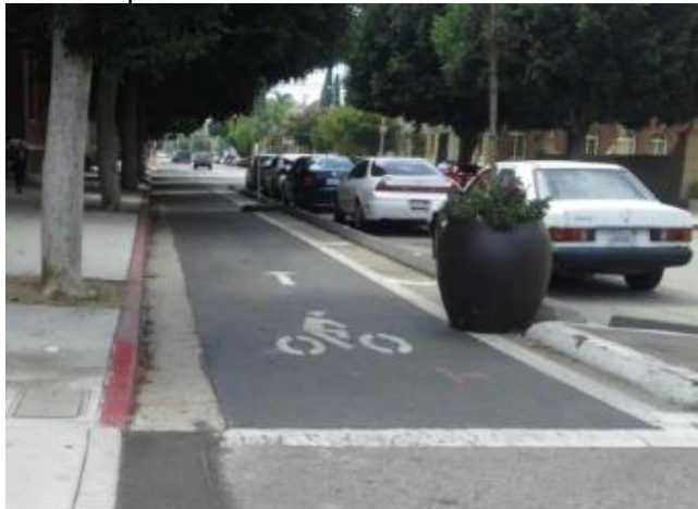
Planter and curb protected
