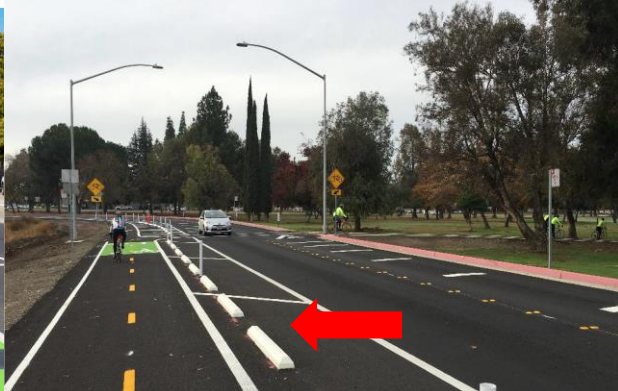
Raised curb and bollard protected
