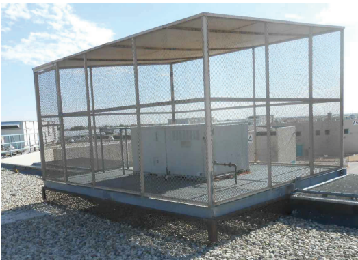
A AC UNIT ON PLATFORM NO SCALE
