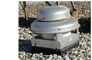
F EXHAUST FAN ON ROOF NO SCALE
