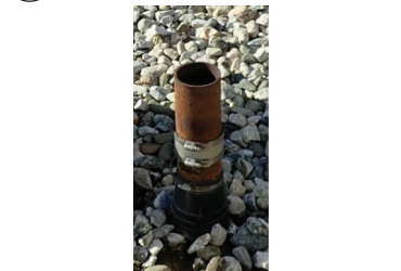
G PLUMBING VENT ON ROOF NO SCALE
