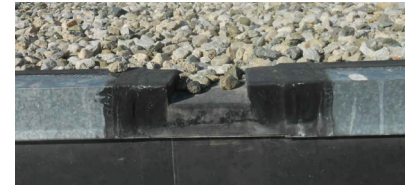
B SCUPPER ON HIGH ROOF NO SCALE
