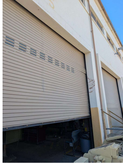
Photo A-2: Roll-up door, exterior view
