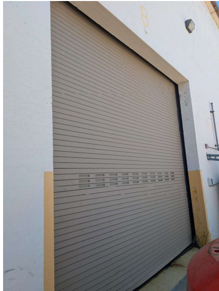
Photo A-3: Roll-up door, Bay 8, exterior view
