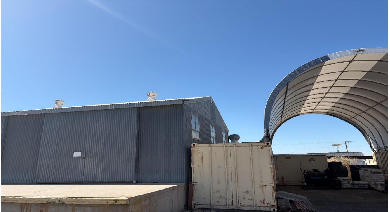
Warehouse_3 ( three windows)
