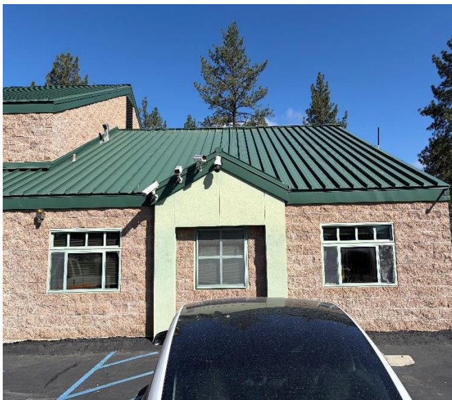
Office_1 (three windows & Screen)
