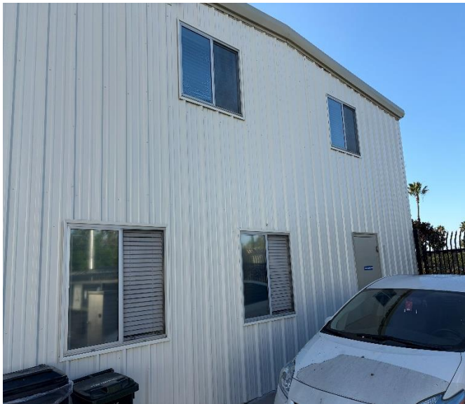
Electrical Office_2 (four windows & screen)
