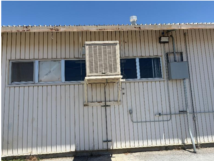
Office/shop_1 ( five windows)
