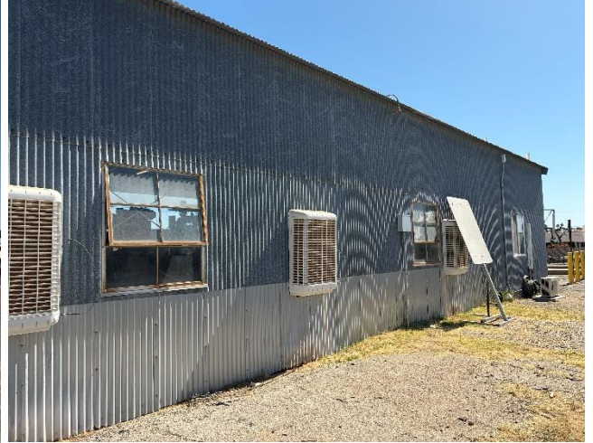
Equipment shop_3 ( two windows)
