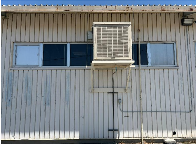
Office/shop_3 (five windows)
