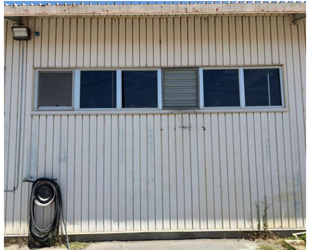
Office/shop_2 ( five windows)
