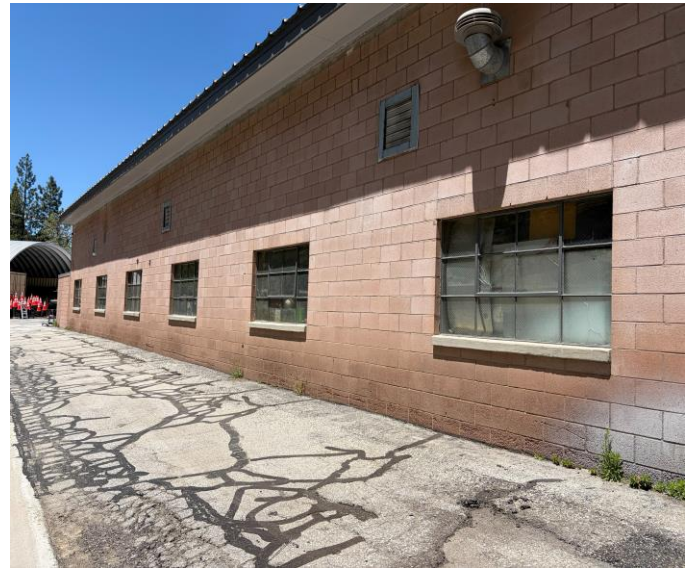
Equipment shop_1 (six windows: no sliding)
