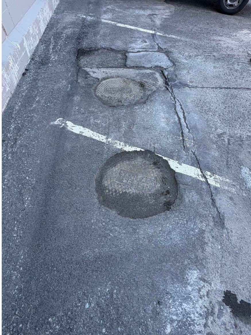
Existing Manholes to be Adjusted to Grade
