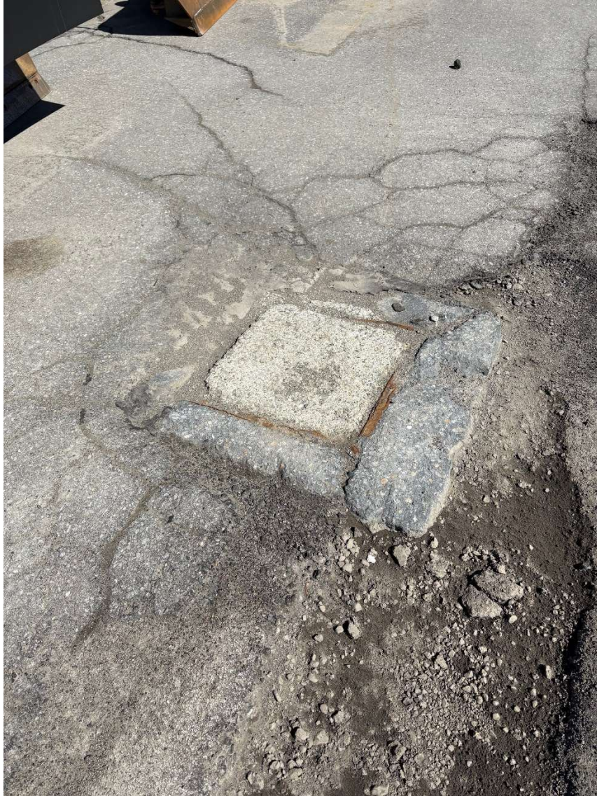
Abandoned 3' x 3' Utility Frame to be Removed
