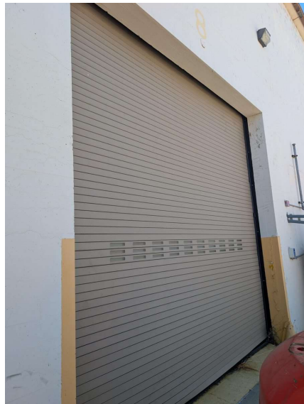
Photo A-3: Roll-up door, Bay 8, exterior view
