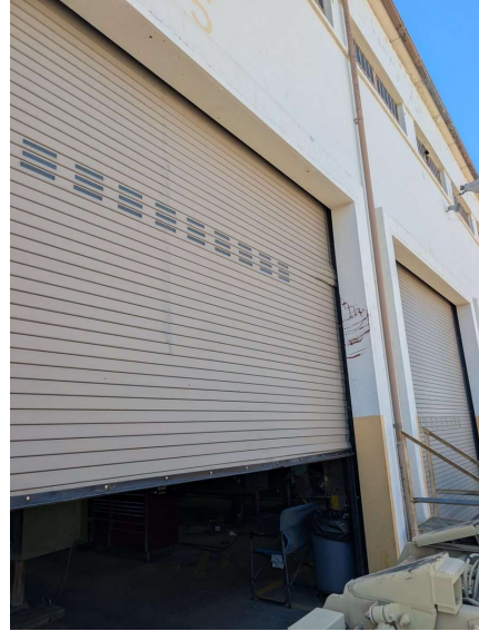
Photo A-2: Roll-up door, exterior view
